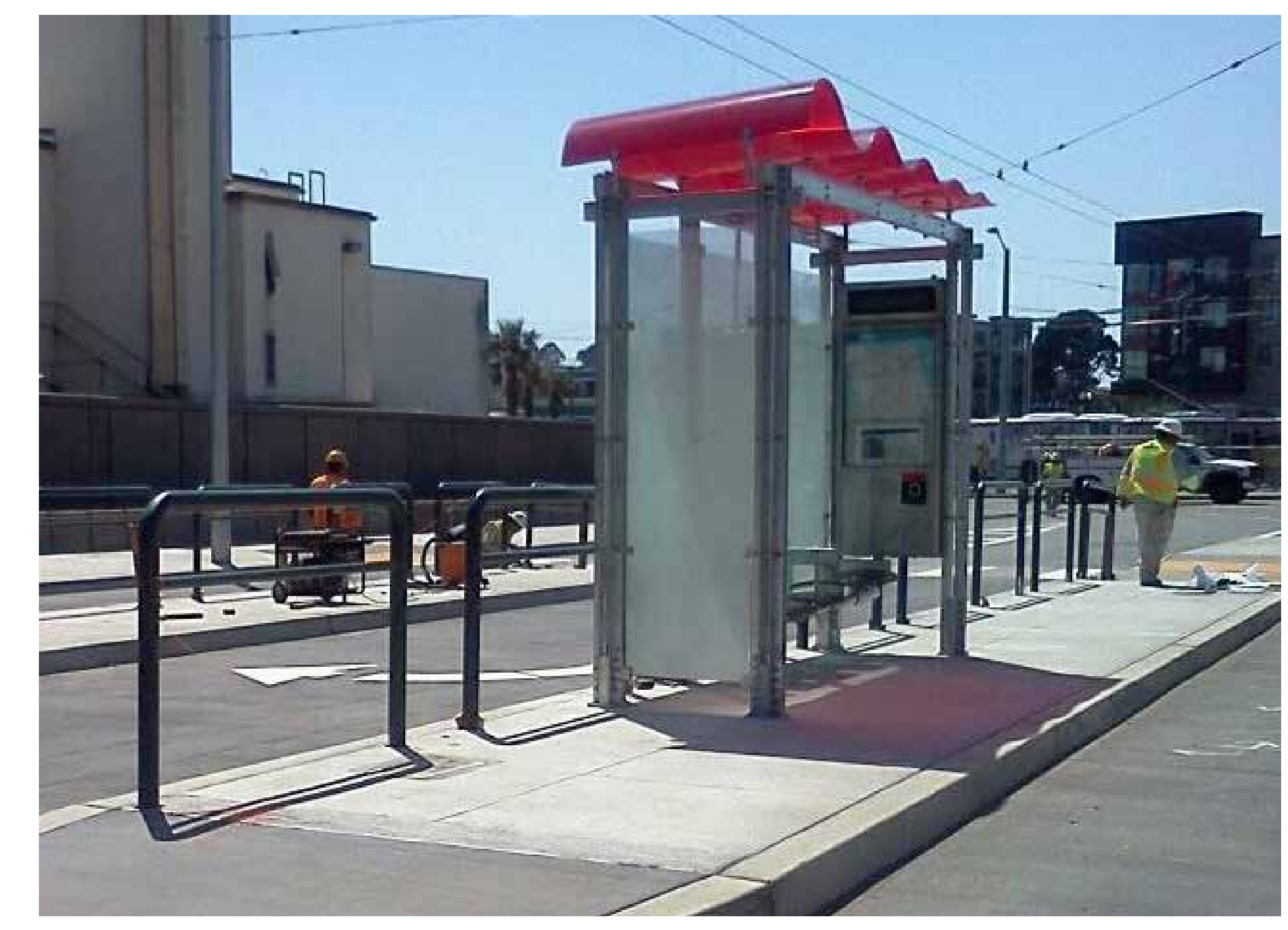
Wide boarding island with upgraded transit shelter
